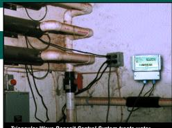
Triangular Wave Deposit Control System treats water before the water enters the UV disinfection units, keeping quartz sleeves clean
